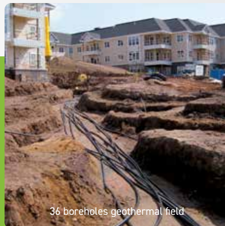
1 ½ TWINLOOP™ waiting for installation
